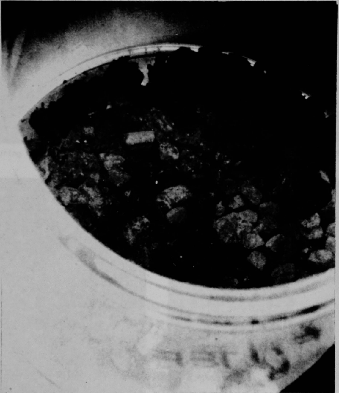
Figure 6. B-loop steam generator tube sheet top loose debris.
